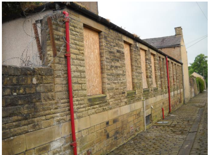
Rear Elevation to Church Back Street
