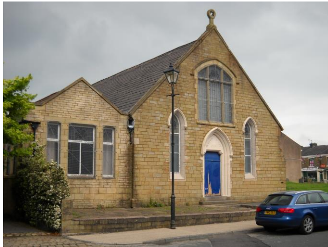
Front Elevation – Existing Building – Church Street
