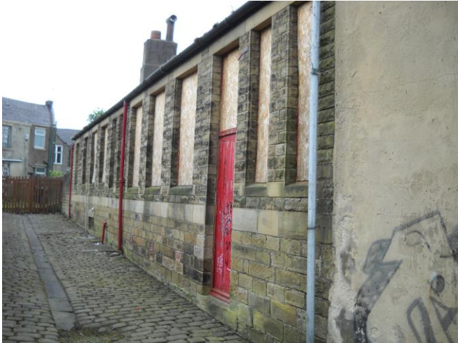
Rear Elevation to back Church Street
